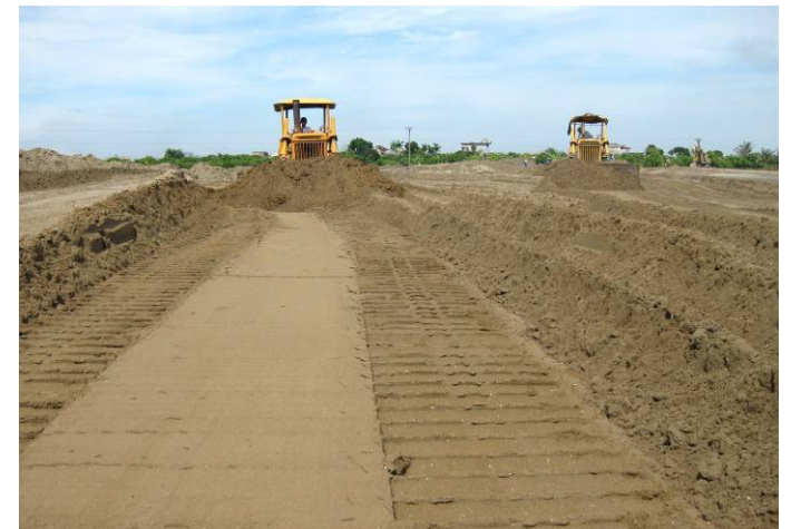
Photo of Hanoi – Hai Phong Highway
